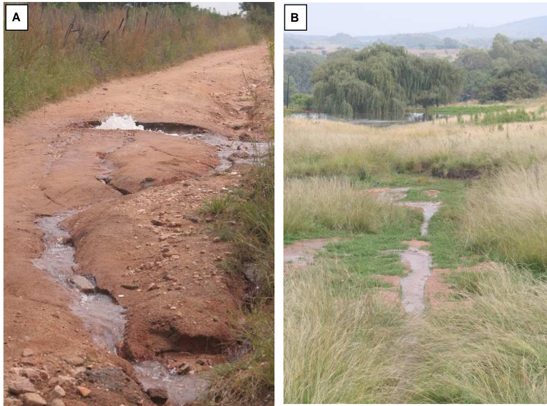
Figure 6: Burst pipe located within study area (A), resulting in channelization of downslope wetland and sediment deposition (B)
